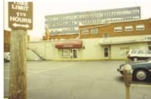
Figure 10.8. Unattractive rear store entrances should be upgraded similar to the bottom photo to make patrons more willing to park behind the building.
