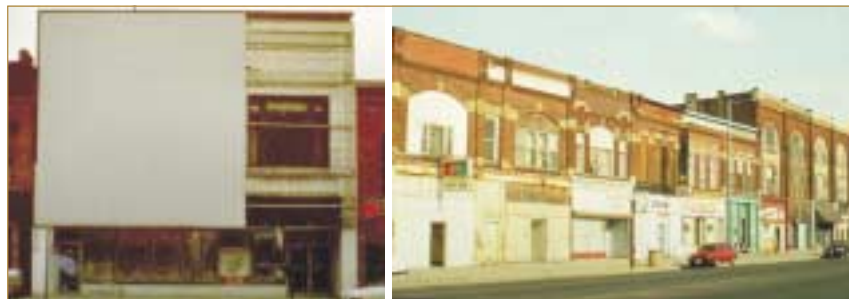
Figure 10.19. Altering building facades severely affects the architectural integrity of unique structures.
